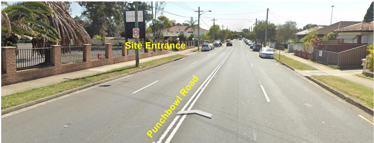
Figure 2-2 Site Entrance from Punchbowl Road looking North (Source: GoogleEarth)
